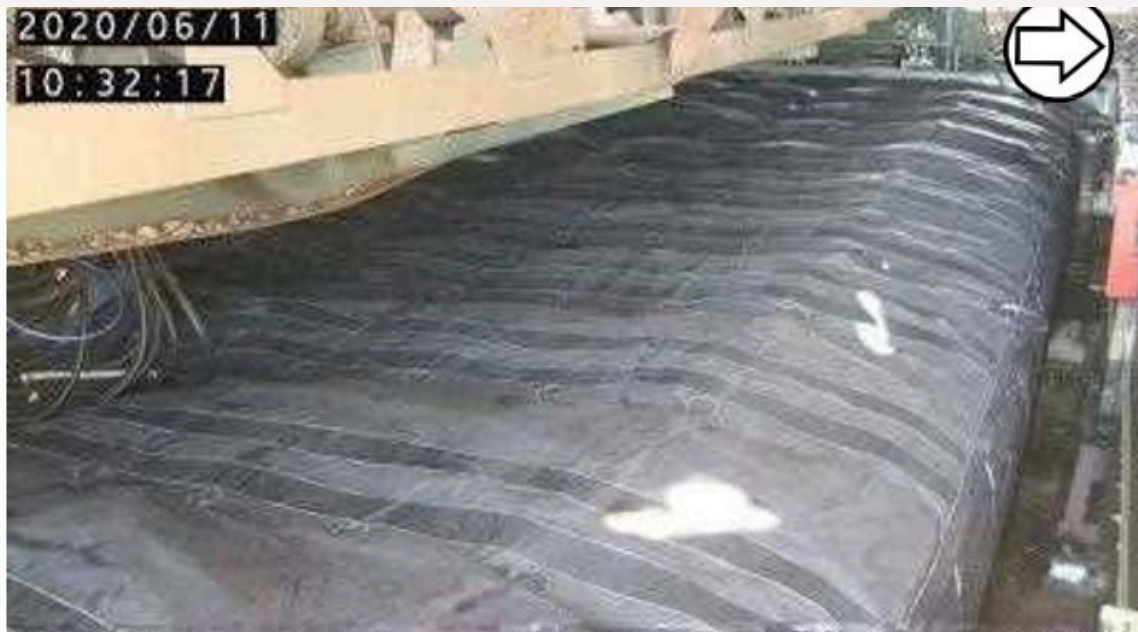
Air mortar filling (Photo date: 2020.6.11)
